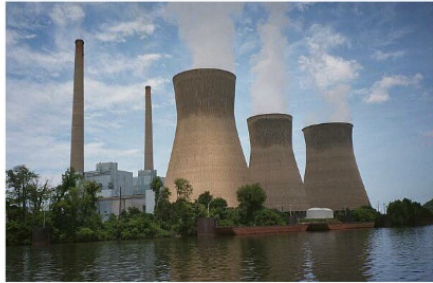
high voltage electricity is produced at the power plant (12 000 V)
